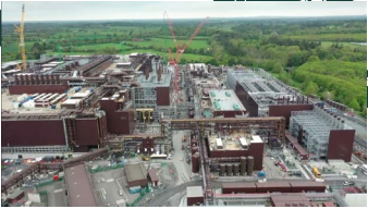
EMEA: 5 fabs under construction, 10 starting operations
